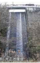
(新)大正池堰堤
